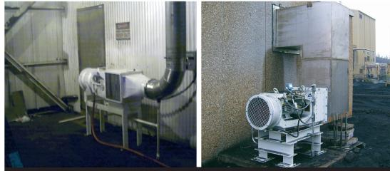
Ambient plant air is pulled into the Englo Extractor by its integrated impeller, cleaned, and then exhausted into the MCC Room.
