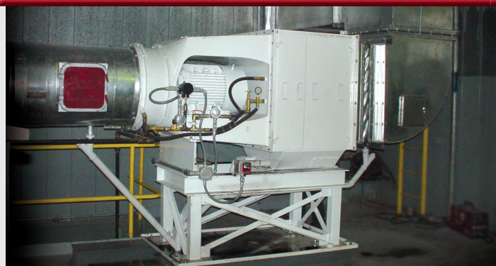
Englo Type 33 - Cascade Conveyor & Silo Ventilation Dust Control
